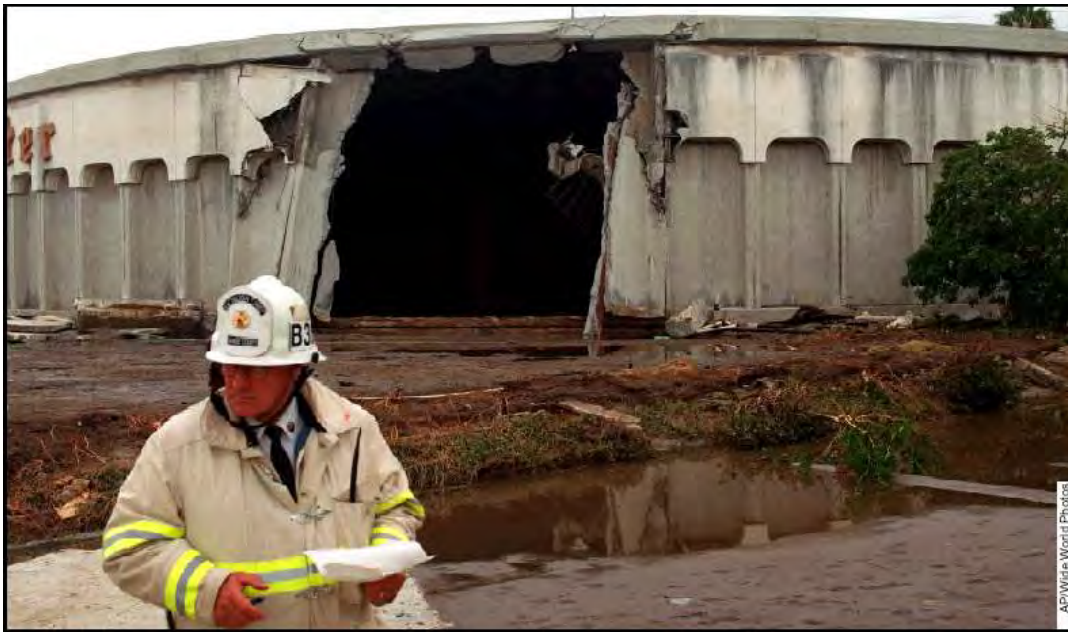
This 31-year-old storage tank ruptured in Westminster, California, sending a 6-foot wave of water through the city that damaged or destroyed about 50 buildings and over a dozen vehicles. Storage tanks should be replaced or periodically rehabilitated to preserve their structural integrity.
