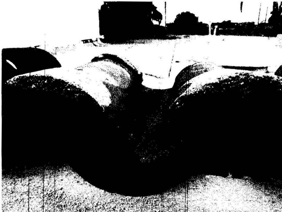
10) Tile has slipped off already – note loose mortar details and missing tile.
