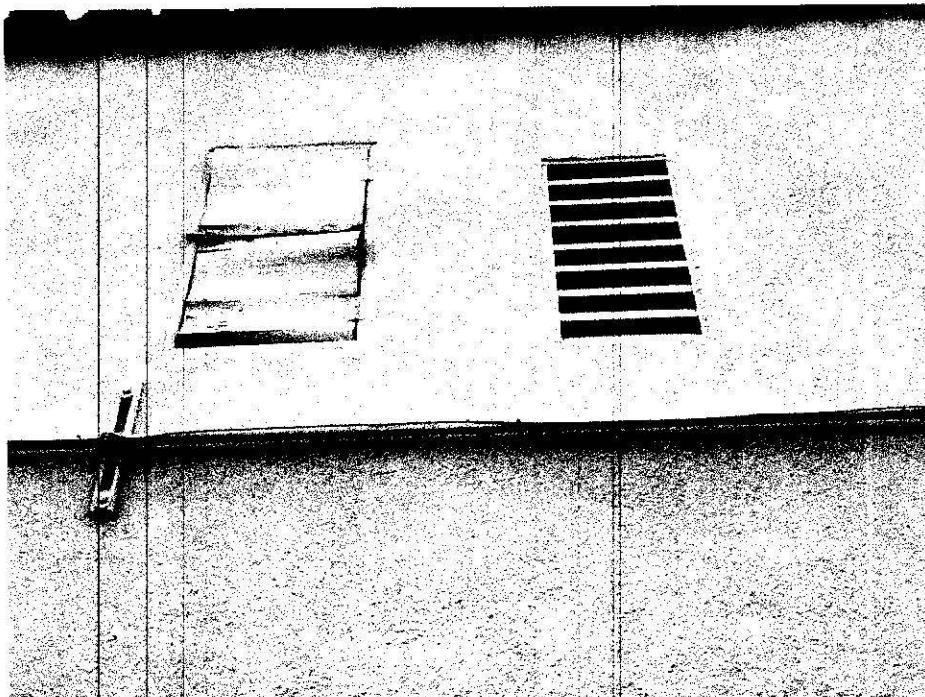
12) Wooden wall panel should be removed and replaced with proper access door.
