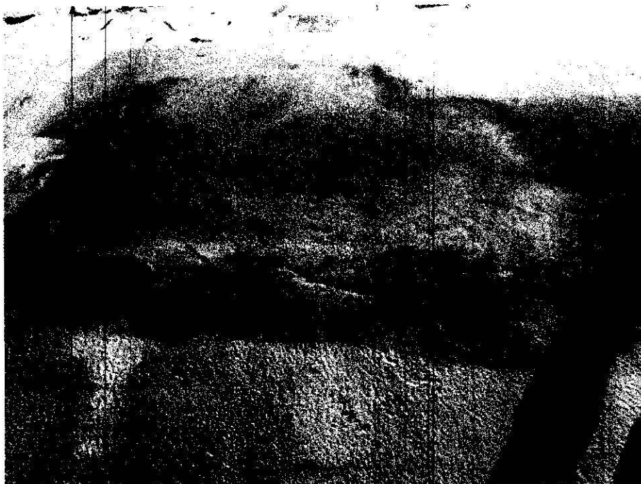
4) Worn roof area due to standing water.
