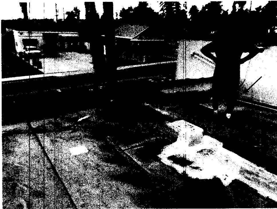
2) Corner drain area needs correcting.
