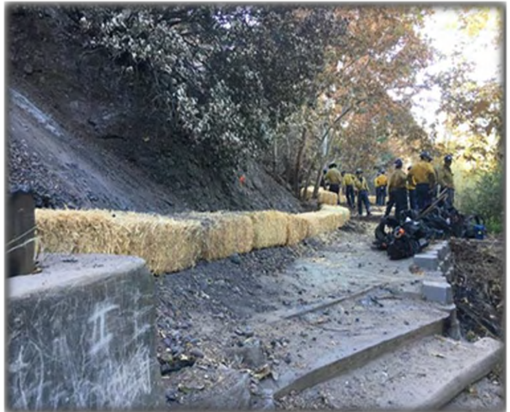
OCFA Hand Crew installed hay bales at the bottom of the slope to control erosion
